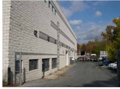
Back of Building
